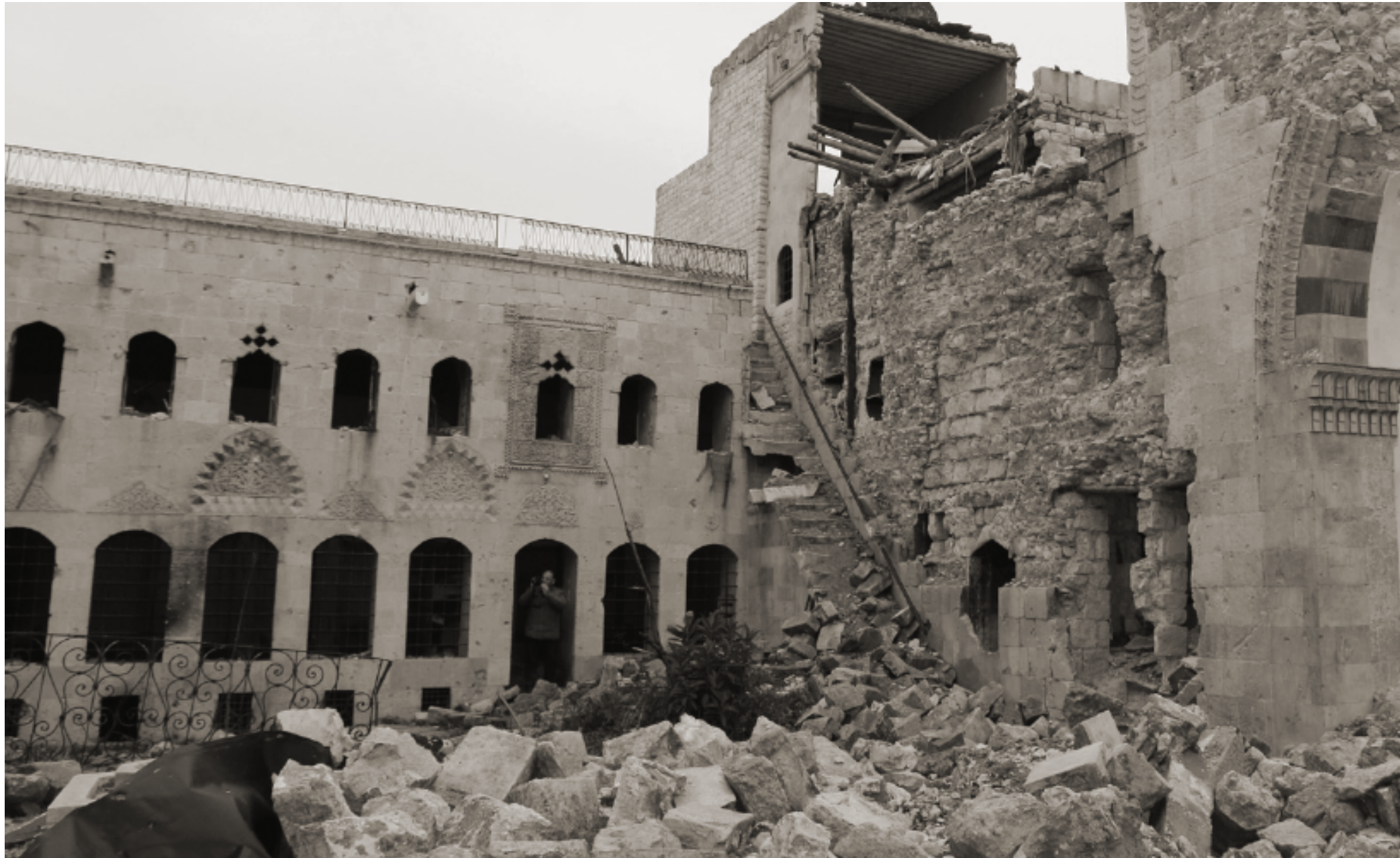
Bayt Ghazaleh, southeastern corner of the residence. Picture date: 16 January 2017 © UNESCO/G.Khawam.
